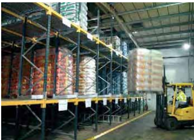
Beam levels at the input face are set at a higher height creating the incline for the pallets.
